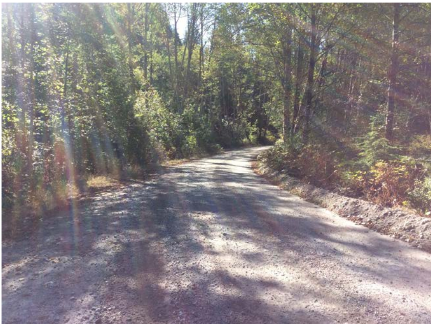
Left approach viewed from bridge
